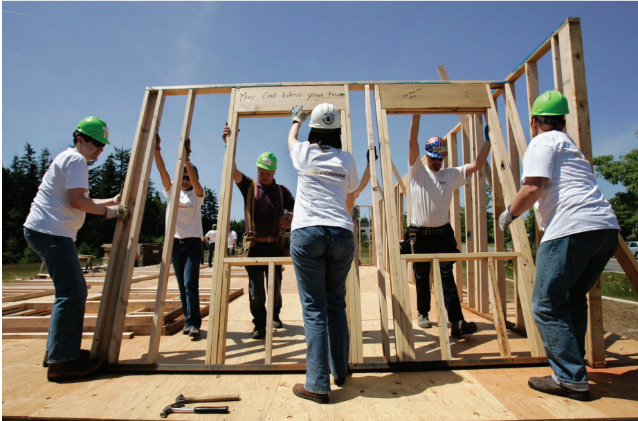
Expedia employees volunteered to quickly build the framework for a Habitat for Humanity house that was shipped to the Katrina-devastated Gulf Coast for a family in need.
