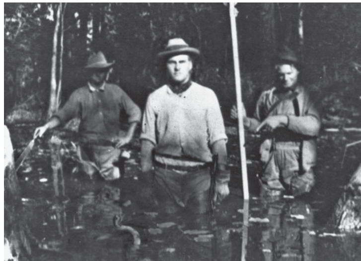
Drainage surveyors in Mississippi County swamps, ca. 1913. Courtesy of Drainage District No. 9, Mississippi County, in Elliott B. Sartain, It Didn't Just Happen (Osceola, Ark.: Grassy Lake and Tyronza Drainage District No. 9, 197?), p. 8.
